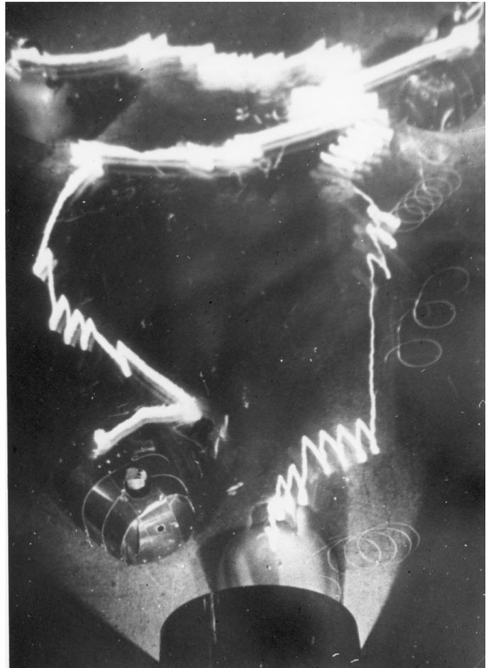
Fig. 4. A time lapse photograph of Elmer and Elsie, taken at Grey Walter’s house in 1949 or 1950, and showing the tortoises interacting with one another. The candles mounted on the backs of the robots trace out their trajectories; the fainter traces are made by the headlamps. Elmer, with the darker segmented shell, starts from the top right, and Elsie from the top left. The hutch is at the bottom of the picture.
